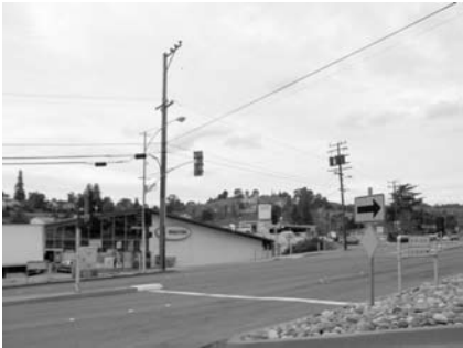
Work with PG&E to underground utilities on major roads in residential neighborhoods, such as here at Lake Chabot Road and Seven Hills.
